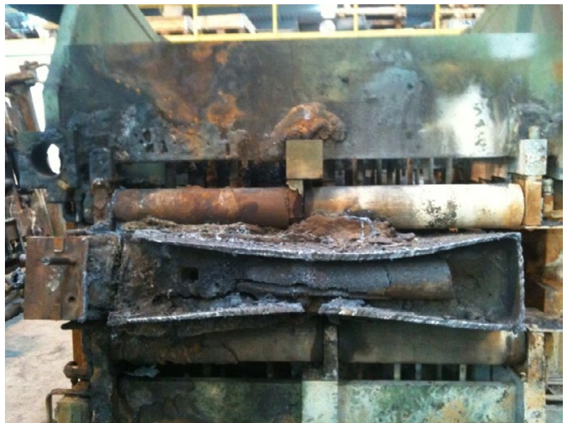
View of a plant breakdown strand looking into the „leaked“ strand
